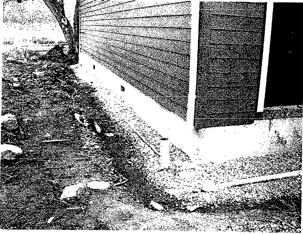
SOUTH SIDE OF BUILDING
