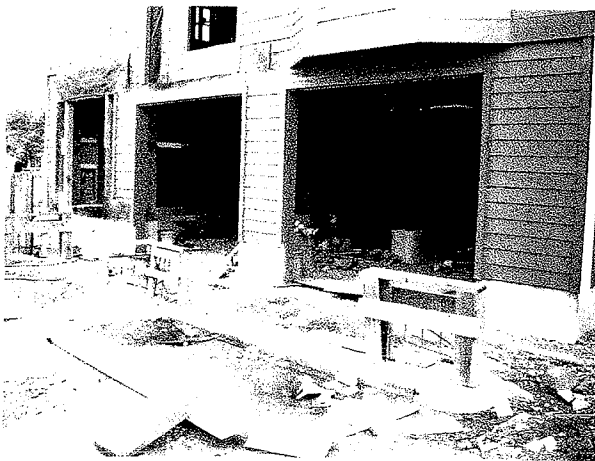
SOUTH SIDE OF BUILDING
