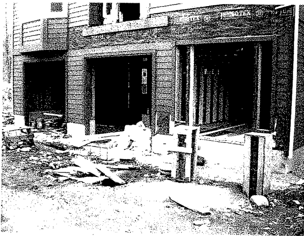
NORTH SIDE OF BUILDING
