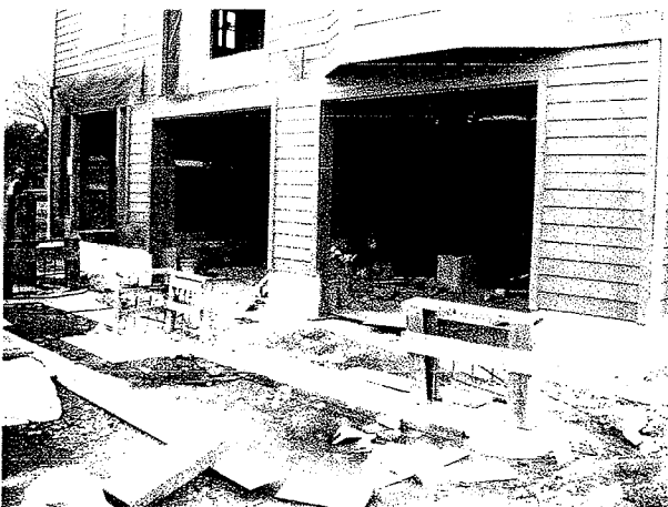
SOUTH SIDE OF BUILDING
