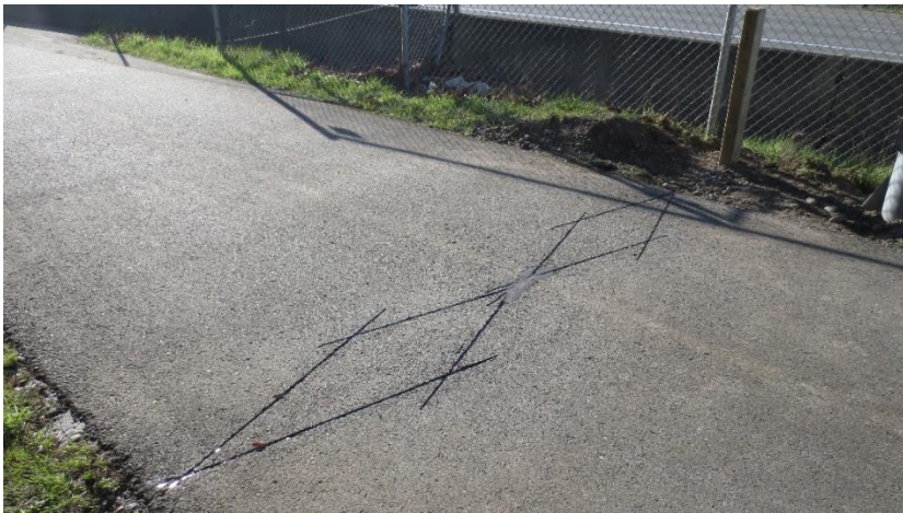
Inductive Loop Detector at SR-520 Trail
