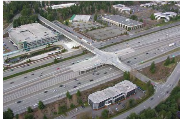
Eastgate Direct Access Ramps
