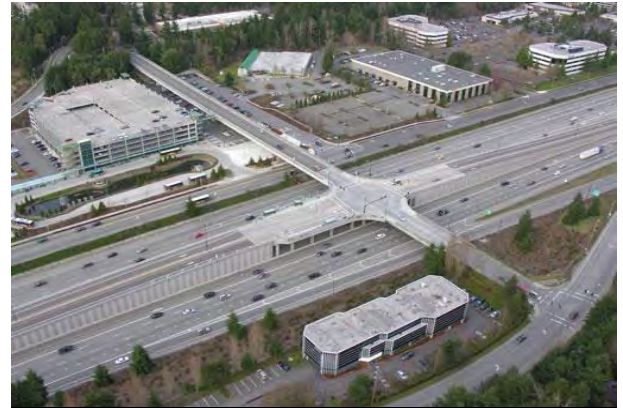
Eastgate Direct Access Ramps
