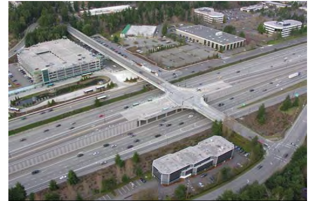
Eastgate Direct Access Ramps
