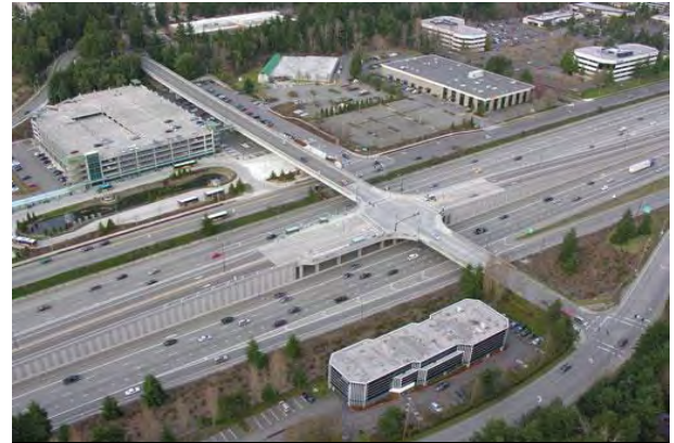
Eastgate Direct Access Ramps
