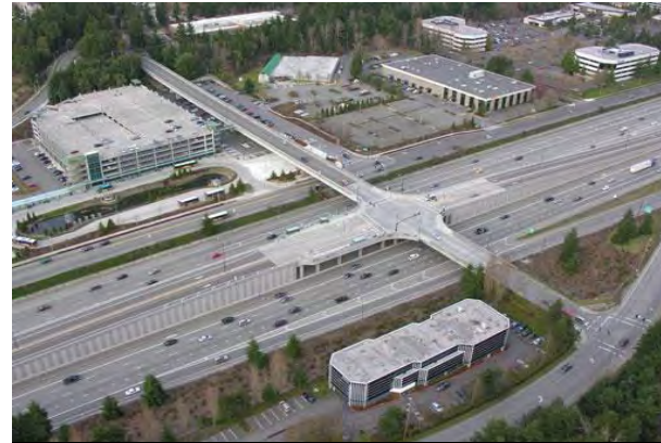
Eastgate Direct Access Ramps
