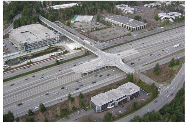
Eastgate Direct Access Ramps
