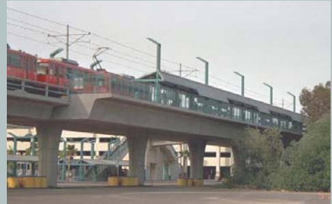
Elevated stations, like this one in San Diego, can be designed to feel safe and welcoming by using high quality materials, lighting, bright stairways, and open architecture. (Source: David Evans and Associates)
