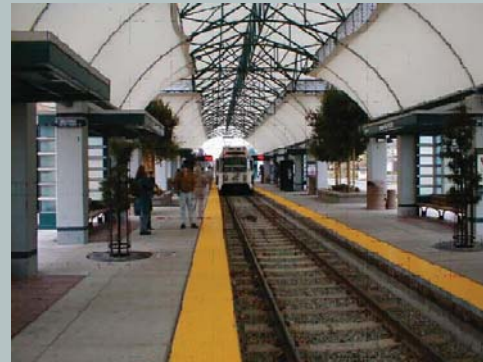
This suburban San Jose station offers protection from weather, while capturing natural light and using open architecture with clear sight lines. (Source: David Evans and Associates)
