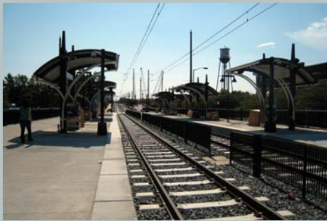
Fences can deter people from running across the tracks, shown here in Charlotte, NC. (Source: Flickr Doug Letterman)
