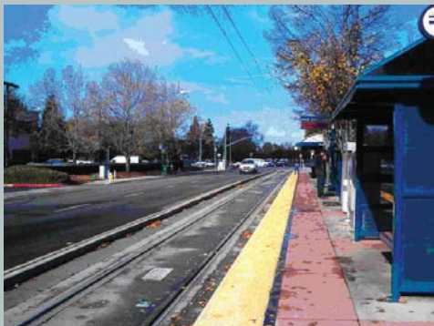
Street configuration and tactile curbs in San Jose. (Source: City of Bellevue)
