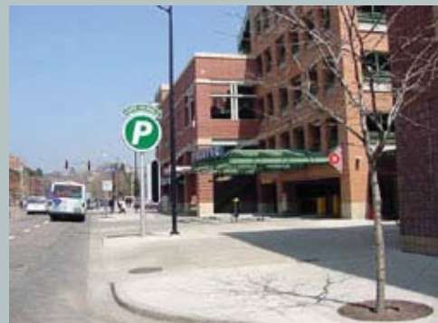
Parking structures in Boulder, CO wrapped in commercial uses and designed to fit into the architectural style of the surrounding area. (Source: David Evans and Associates)
