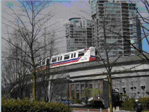
Elevated trackway in Vancouver, B.C. (Source: David Evans and Associates)
