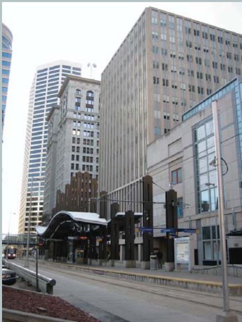
An at-grade light rail station in Minneapolis, MN. (Source: David Evans and Associates)
