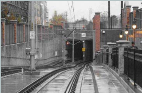
Urban tunnel portal in San Jose, CA. (Source: David Evans and Associates)
