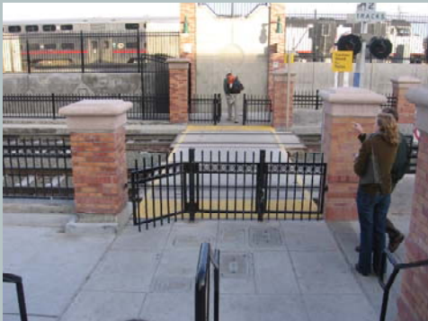
Pedestrian gates force pedestrians to slow down and be aware of trains while crossing the trackway. (Source: David Evans & Associates)
