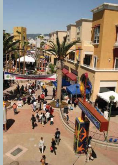
Fruitvale Station in Oakland, CA is a redevelopment project on a commercial strip near a Bay Area Rapid Transit station that includes retail, office, and housing elements. (Source: David Evans and Associates)
