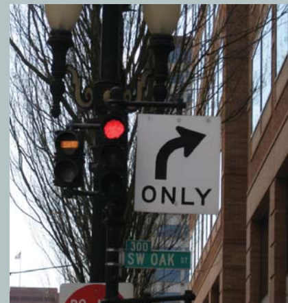
Distinct signals for light rail trains reduce confusion for motorists and help to prevent collisions. The horizontal light bar on the left is for light rail trains; the standard street signal on the right is for other vehicles. (Source: David Evans & Associates)
