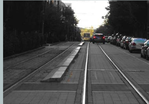
Exclusive and shared use trackway delineation in Jersey City, NJ. (Source: David Evans and Associates)
