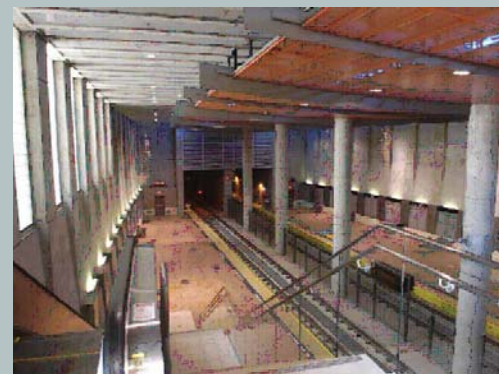
The San Diego State University tunnel employs design features including natural light and air, high quality finishes, and art to create a comfortable waiting environment. (Source: David Evans and Associates)
