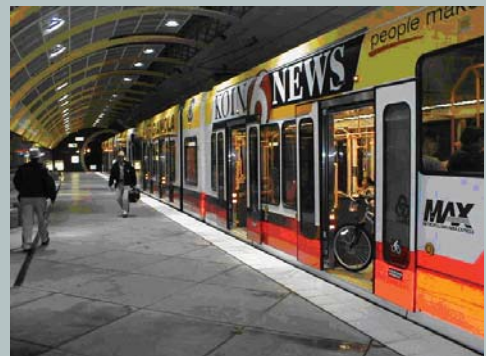
Underground station serving two-car light rail trains in Portland, OR. (Source: David Evans and Associates)
