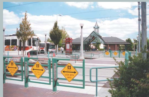
Pedestrian safety gates at Beaverton Transit Center, a busy station serving buses and light rail. (Source: David Evans and Associates)
