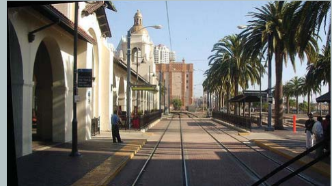
This San Diego station uses architectural detailing that is consistent with the surrounding community, complementing the area’s established identity. (Source: David Evans and Associates)
