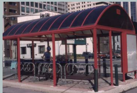
Bike parking at stations should be protected from poor weather and in plain view to prevent theft -- note glass enclosure above. (Source: David Evans and Associates)
