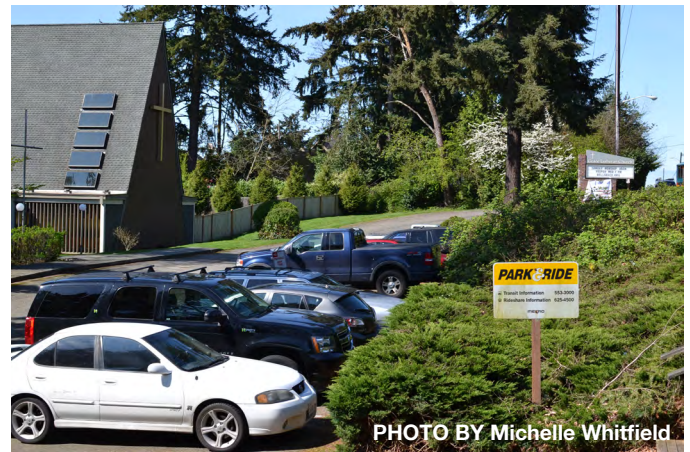
Figure 78 Grace Lutheran Church on NE 8th St and 96th Ave NE serves as a leased park-and-ride lot on weekdays, providing access to Route 271 just west of Downtown.
