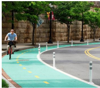
Paint & Delineator Posts
