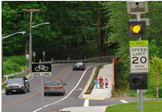
School Zone Flashing Beacon
