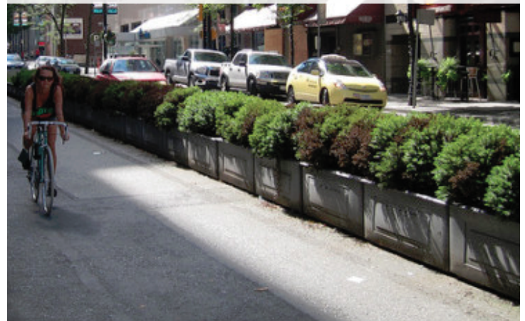
Planter Box Protected Bike Lane
